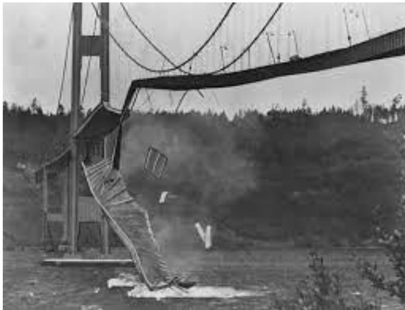
Fig 1 - Flow induced vibration caused the Tacoma Narrows Bridge to experience vertical and torsional vibrations leading to its collapse 1940 [1]
